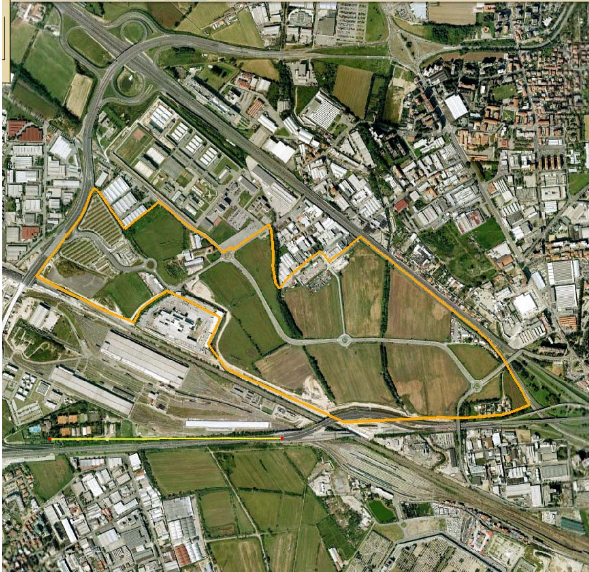
Aerial picture of the area of local pilot application
